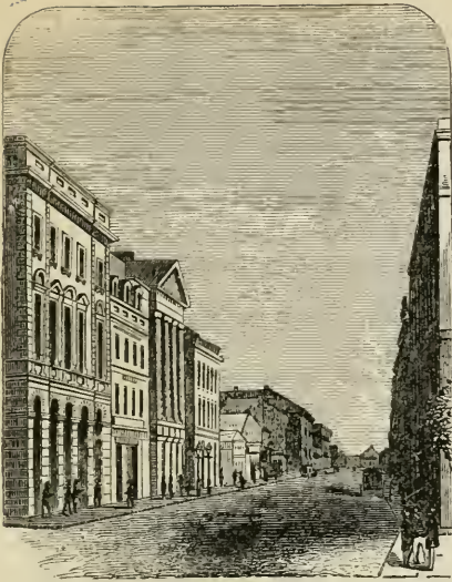
SOUTH SIDE OF GREAT ST. JAMES' STREET.
